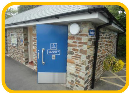
Priory Road Carpark, St Austell
